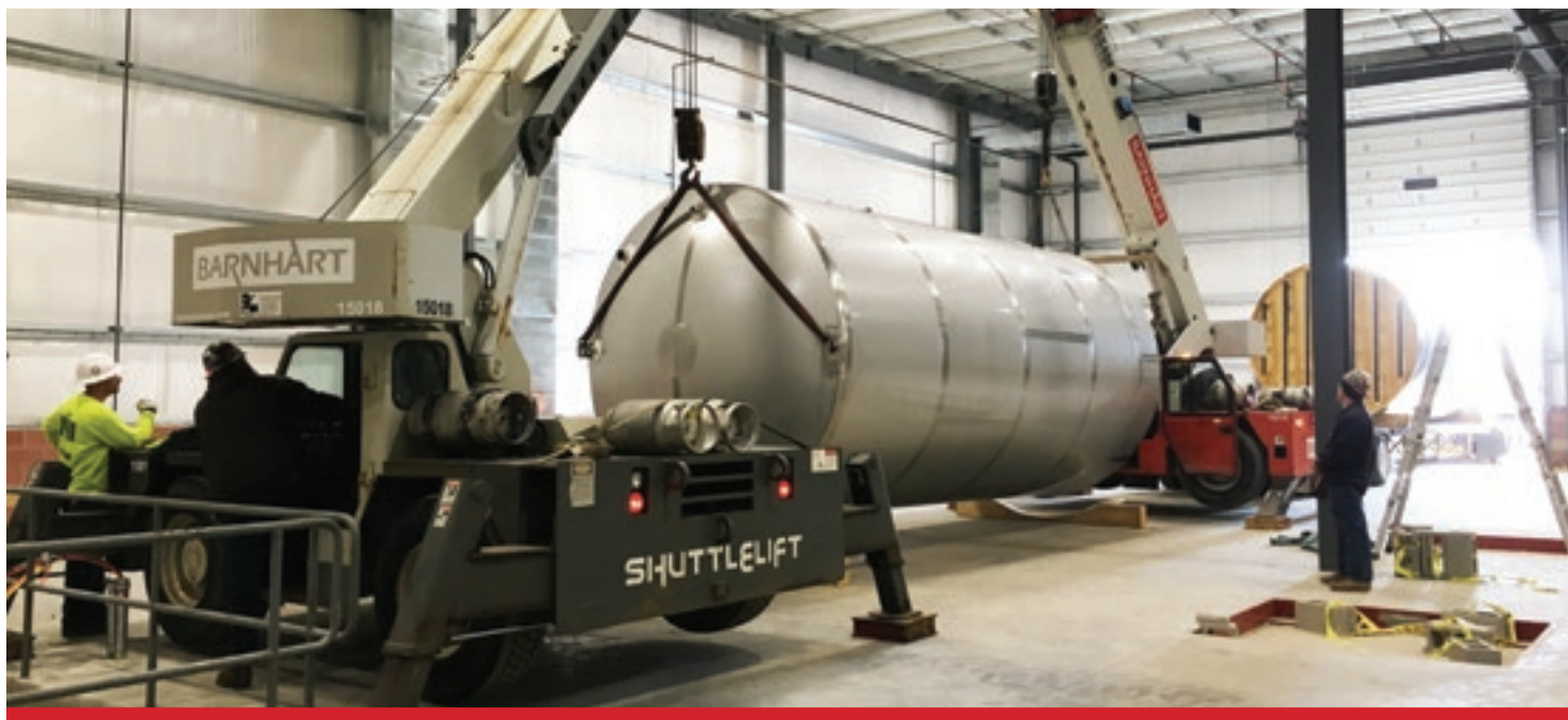
UNLOADING AND SETTING VESSELS INTO A PIT WITH LOW HEADROOM IN A CUSTOMER'S BUILDING.
