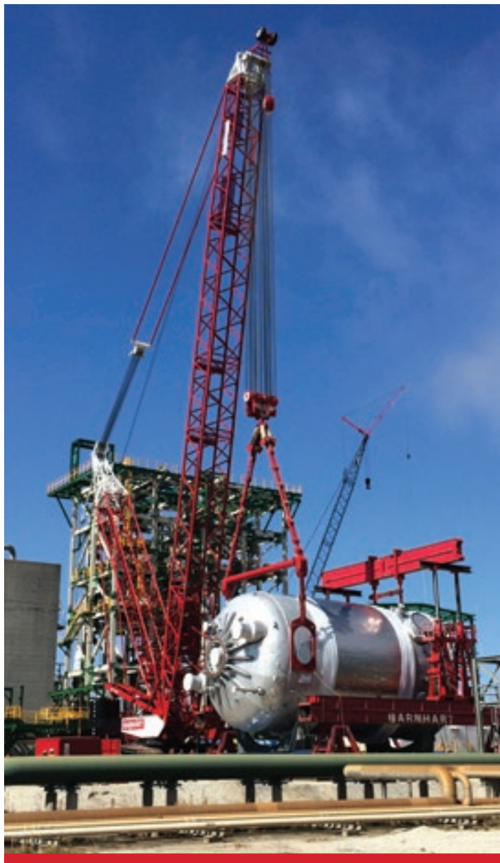
UNLOADING THE REACTOR USING THE ADJUSTABLE LINK RIGGING SYSTEM BEING TAILED WITH 500-TON GANTRIES.
