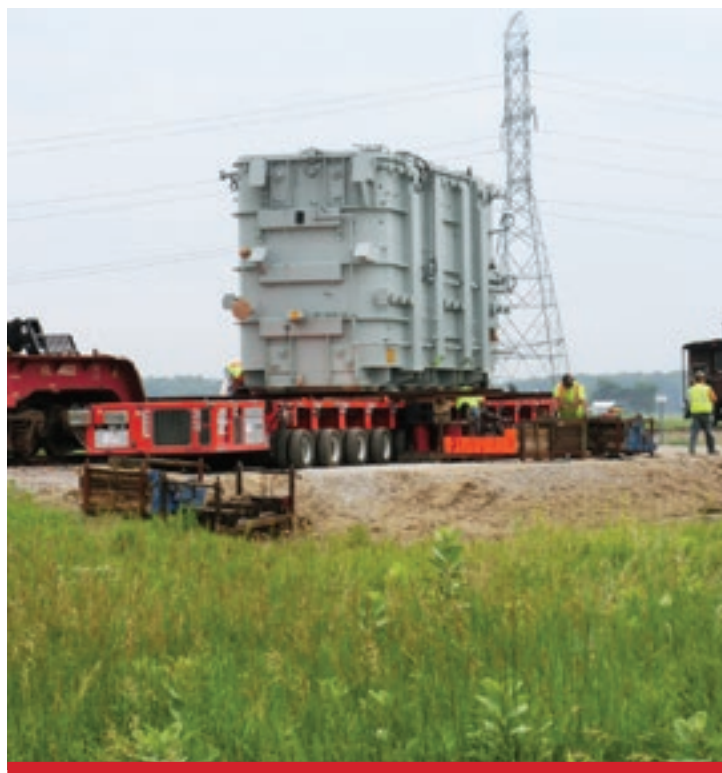
TRANSLOADING, HAULING, AND SETTING A 300,000-POUND TRANSFORMER IN INDIANA.
