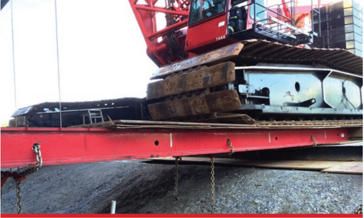
THE BEAMS BRIDGING OVER THE DUCTWORK.
