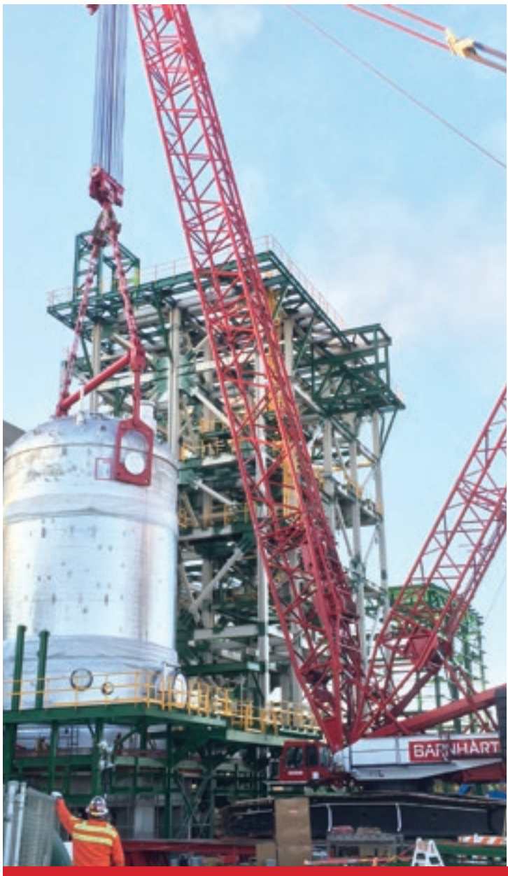
THE REACTOR BEING SET IN ITS FINAL POSITION.
